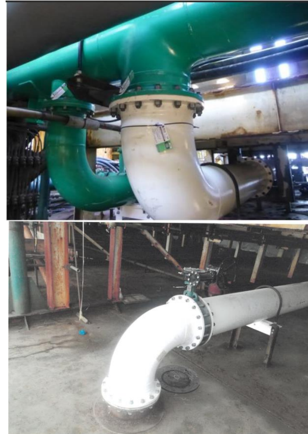
Pipe replacement on Triton FPSO
